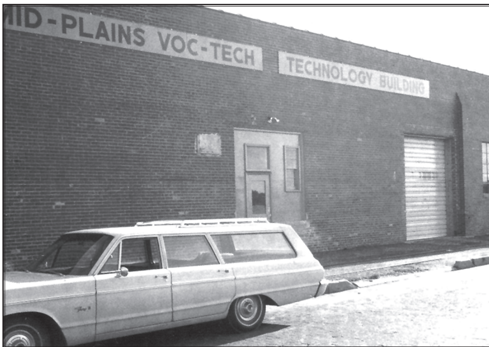
Welding, Machine Shop and Building Construction Entrance
