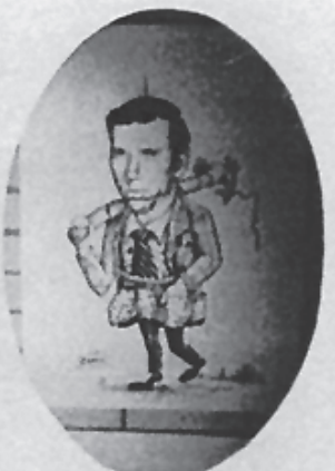
Charles Suiter Building Construction
