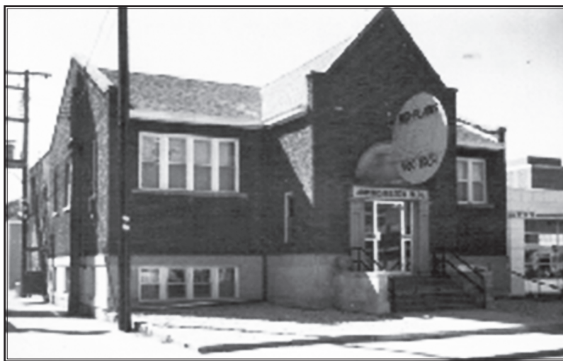
Administrative Building Main Entrance
